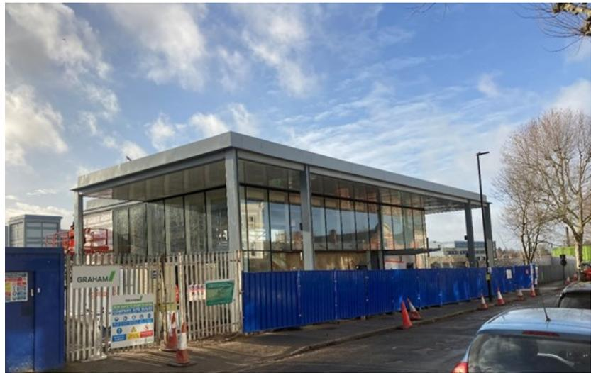
Over the last month we have completed the installation of the external doors and glazing at **West Ealing** and are close to completing the installation of the new concourse ceiling. We have
